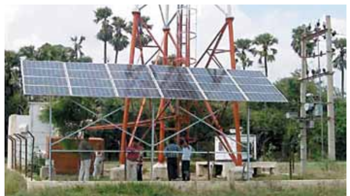
Infratel's 6 mega watt solar installation on the Airtel tower network is India's largest.
